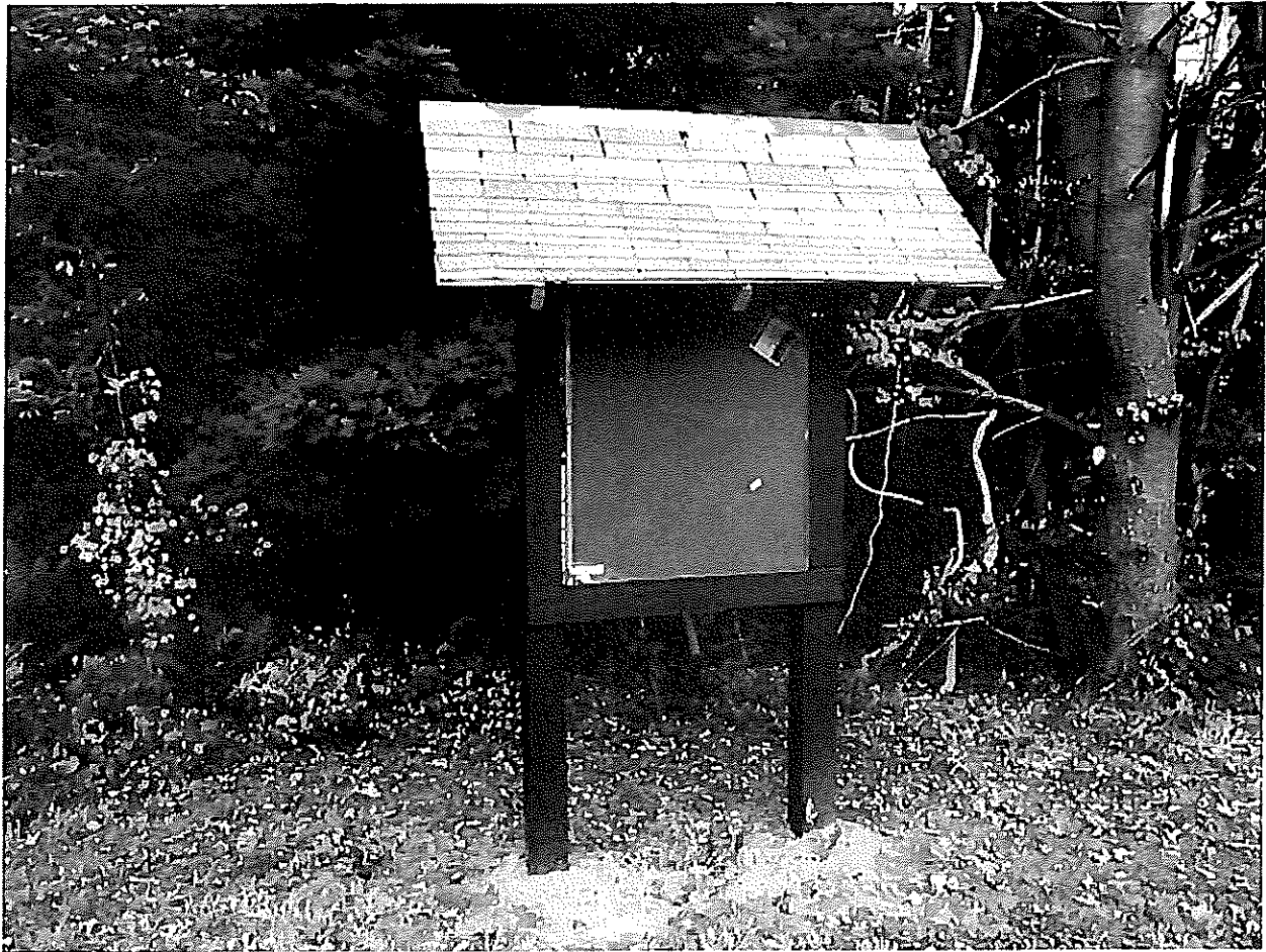
Pinnacle Kiosk constructed by Eagle Scout Justin Taylor
